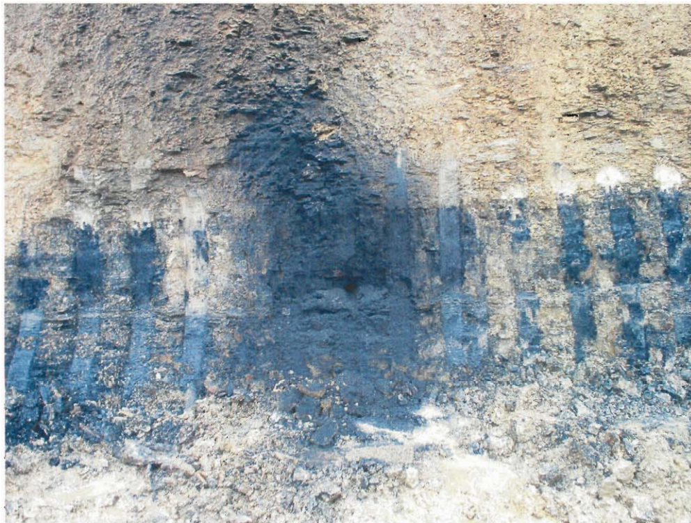
Photograph 20 Source Hole After Blast
