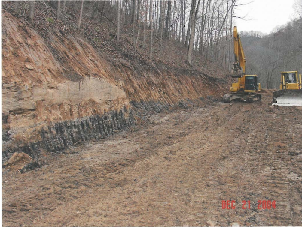
Photograph 11 Exposing the Coal Seam
