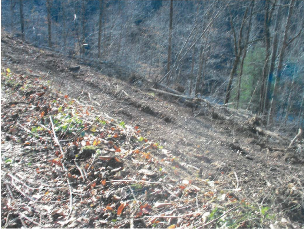
Photograph 3 Access Road Prepared First
