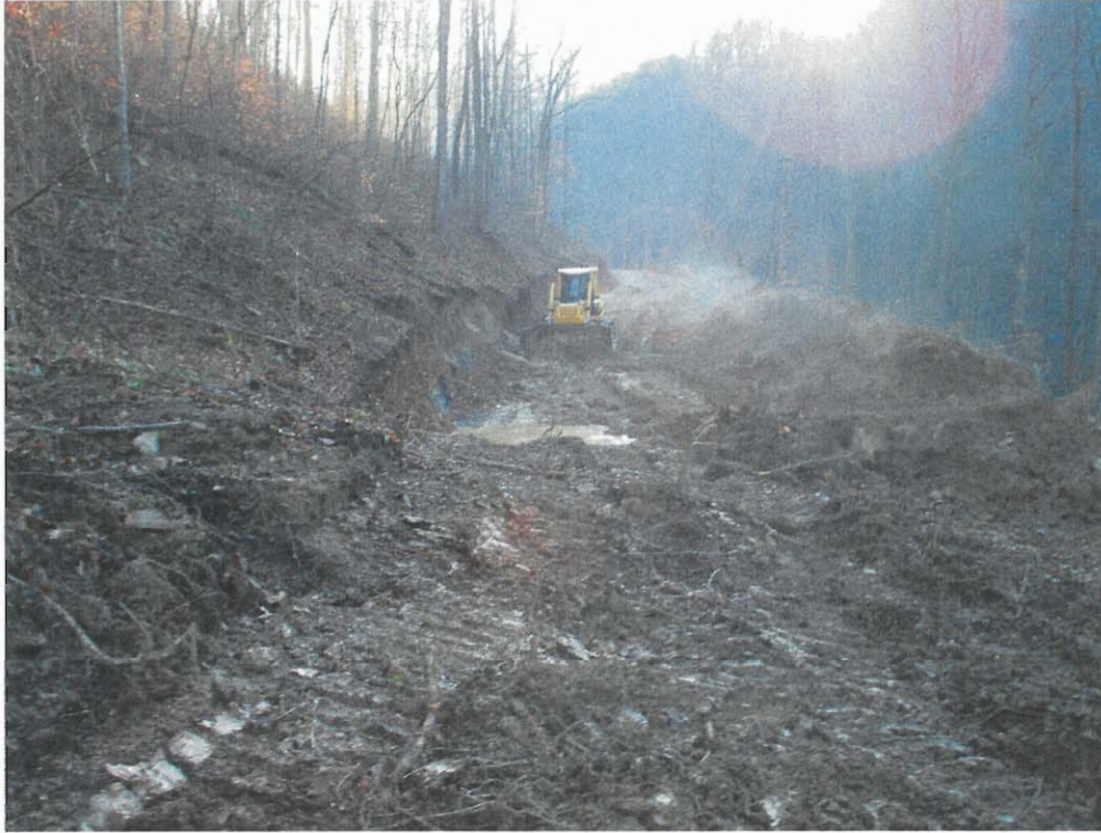
Photograph 5 Exposing the Coal Seam
