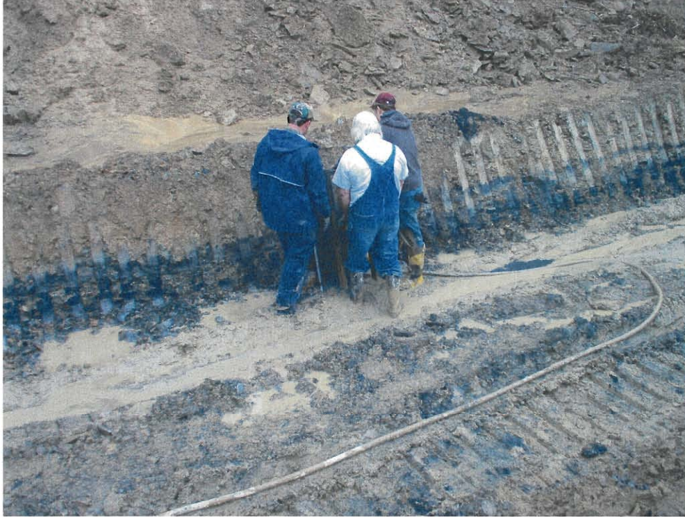
Photograph 17 Drilling Blast Holes
