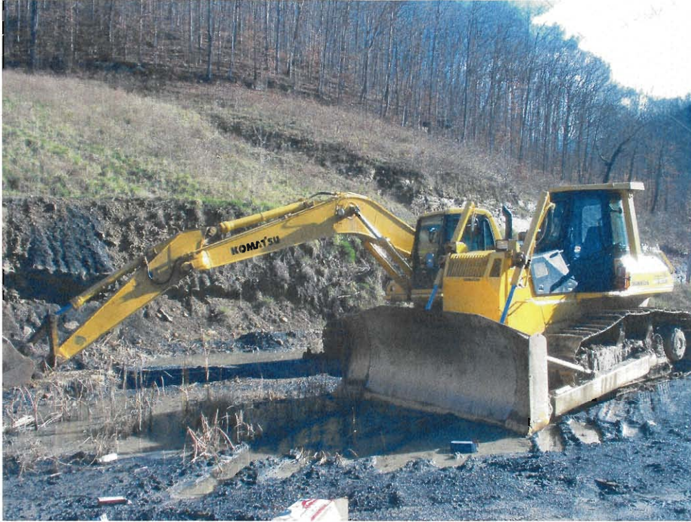
Photograph 1 Equipment Used for Site Preparation
