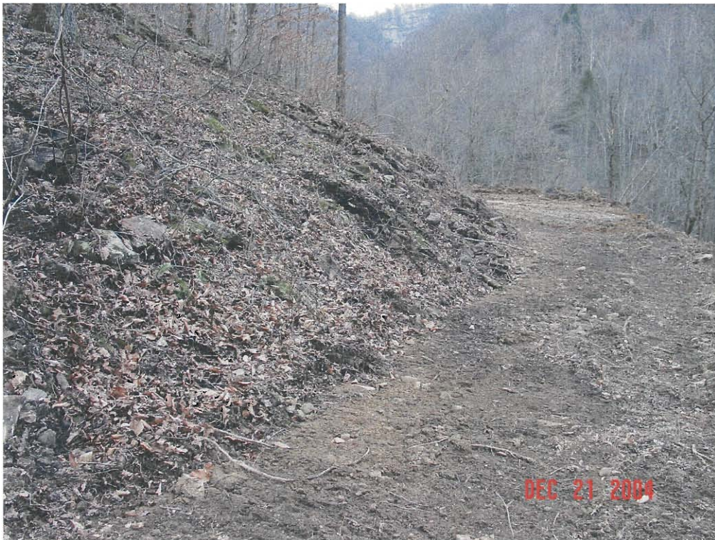
Photograph 4 Site Ready for Coal Seam Exposure
