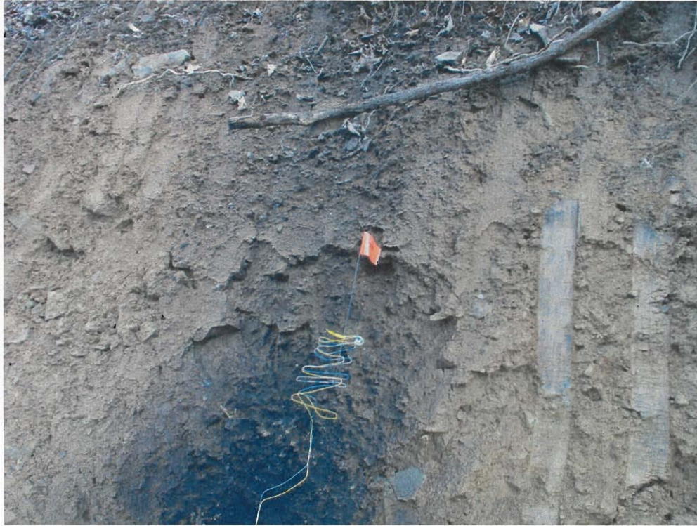
Photograph 19 Blast Hole (Source) Wired and Ready
