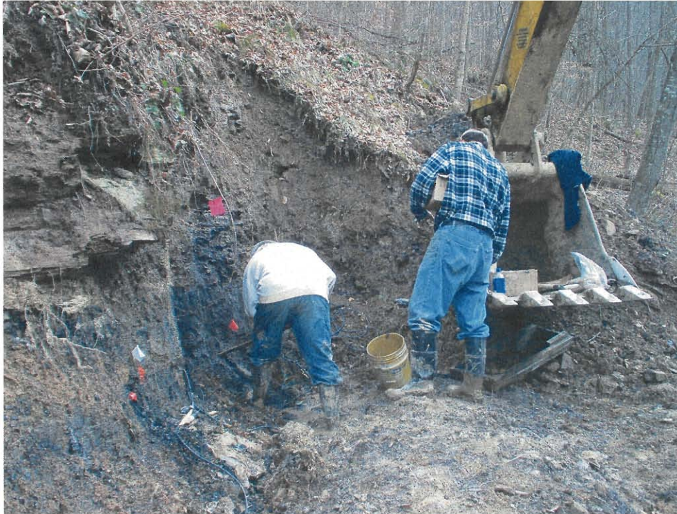
Photograph 18 Placing Charge
