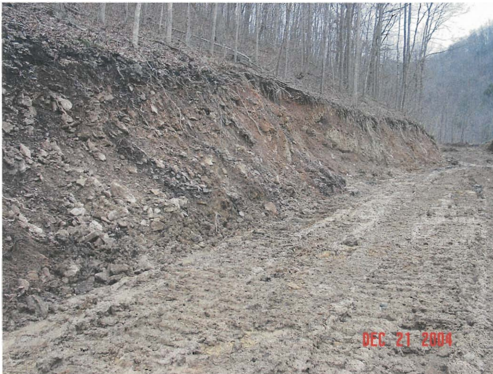
Photograph 8 Exposing the Coal Seam
