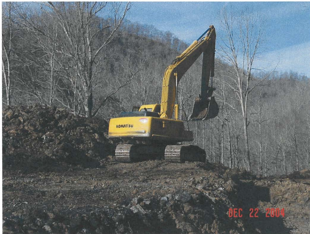
Photograph 16 Preparing the Site
