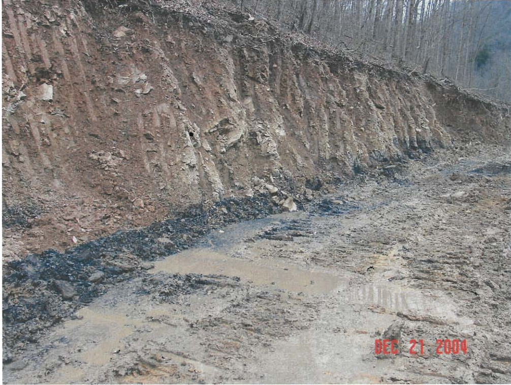
Photograph 9 Exposing the Coal Seam
