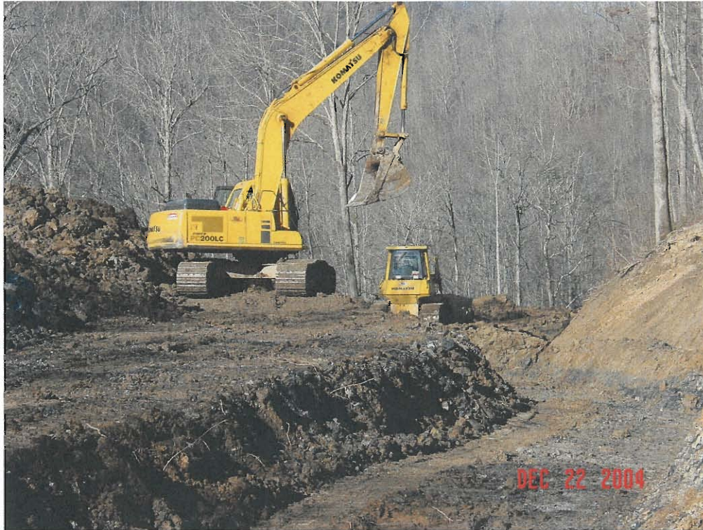
Photograph 15 Preparing the Site
