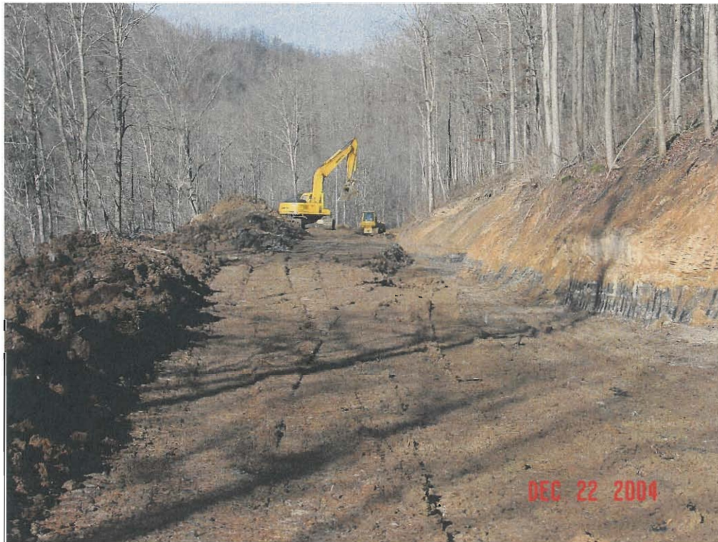
Photograph 14 Preparing the Site
